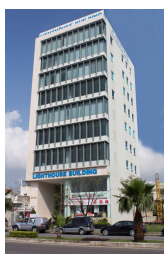
Lighthouse building Đà Nẵng
